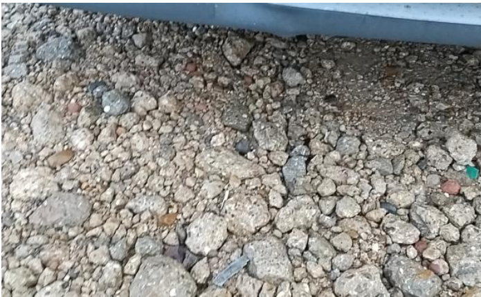
3: Screen Front Chipped UpTo 10mm
