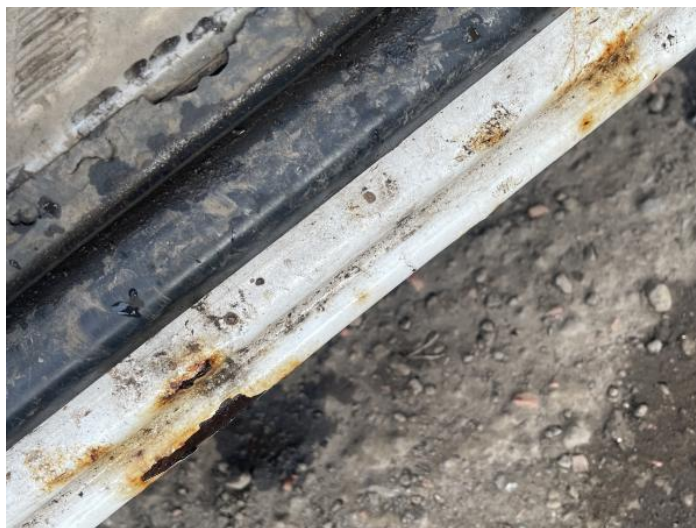
2: Sill os Rusted Over 5mm
